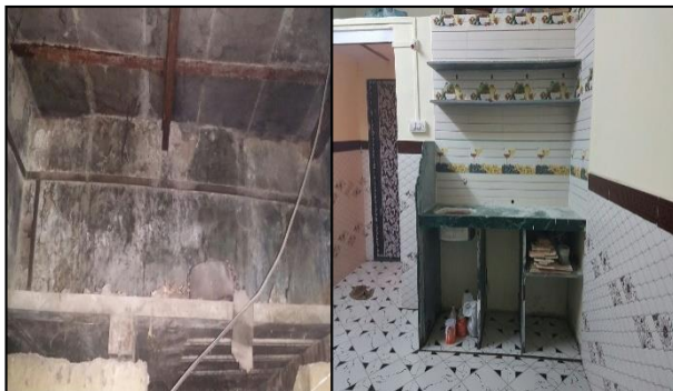
House repair projects
